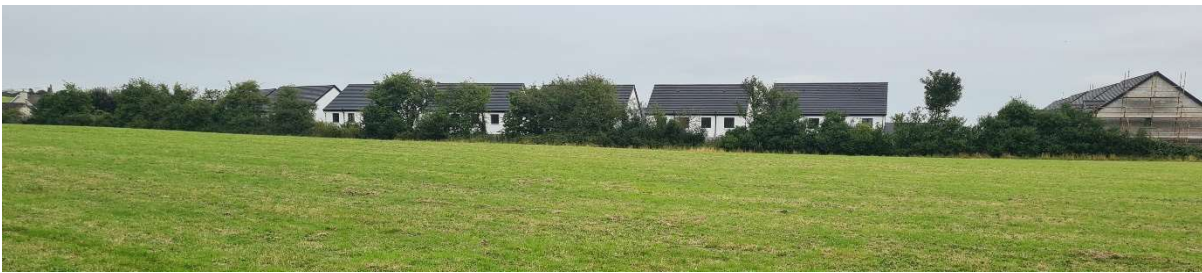
Looking east on to the existing hedgerow between the development site and Hazelbrooke where construction is more advanced.
