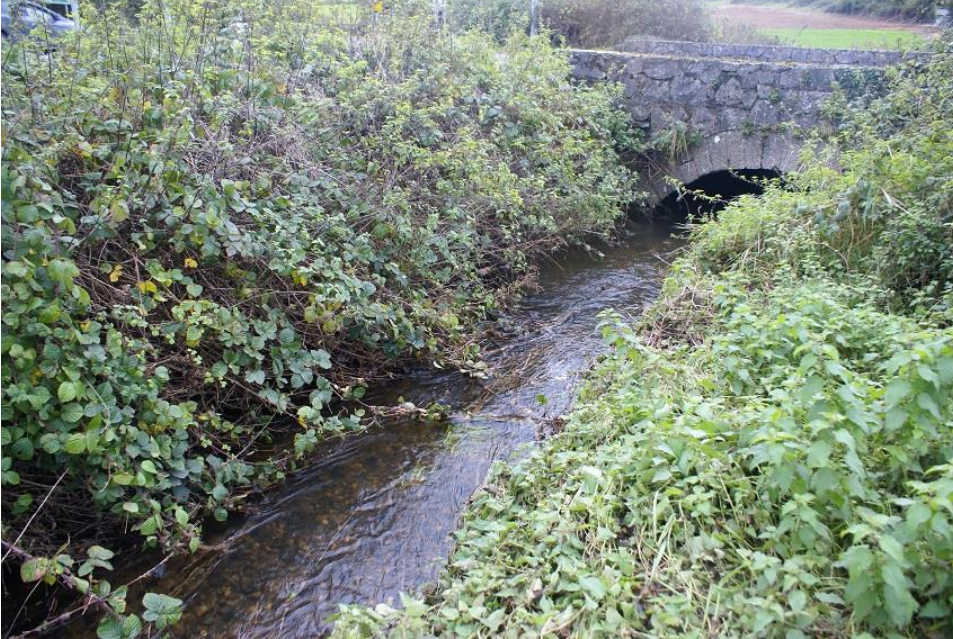
Photo 3: Downstream end of Spa Glen Stream within subject site
