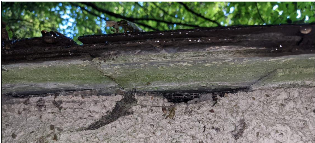
Plate 3-1: Visible gap in the farm stable roof
