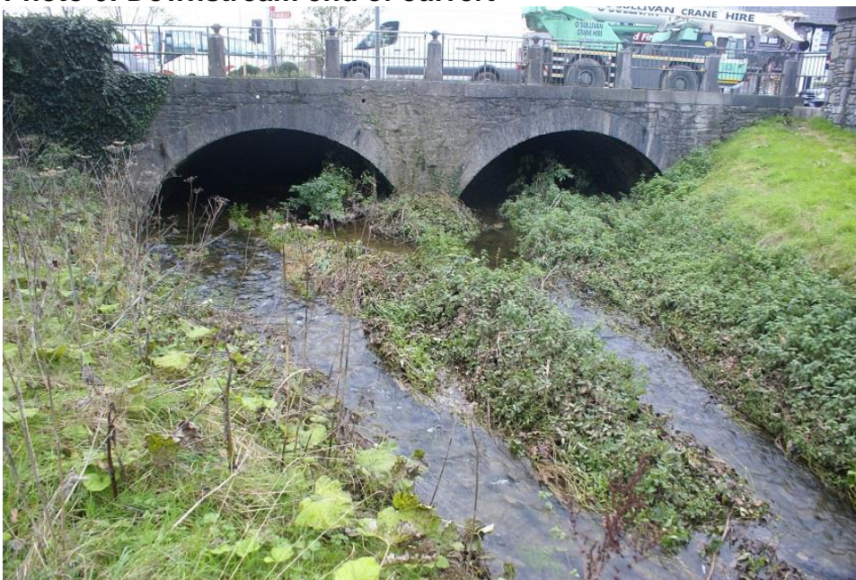
Photo 6: Downstream end of culvert
