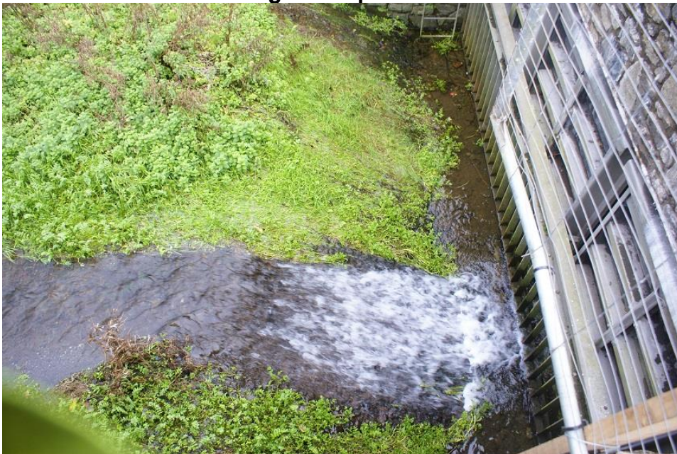
Photo 5: Weir and metal grid at upstream end of culvert
