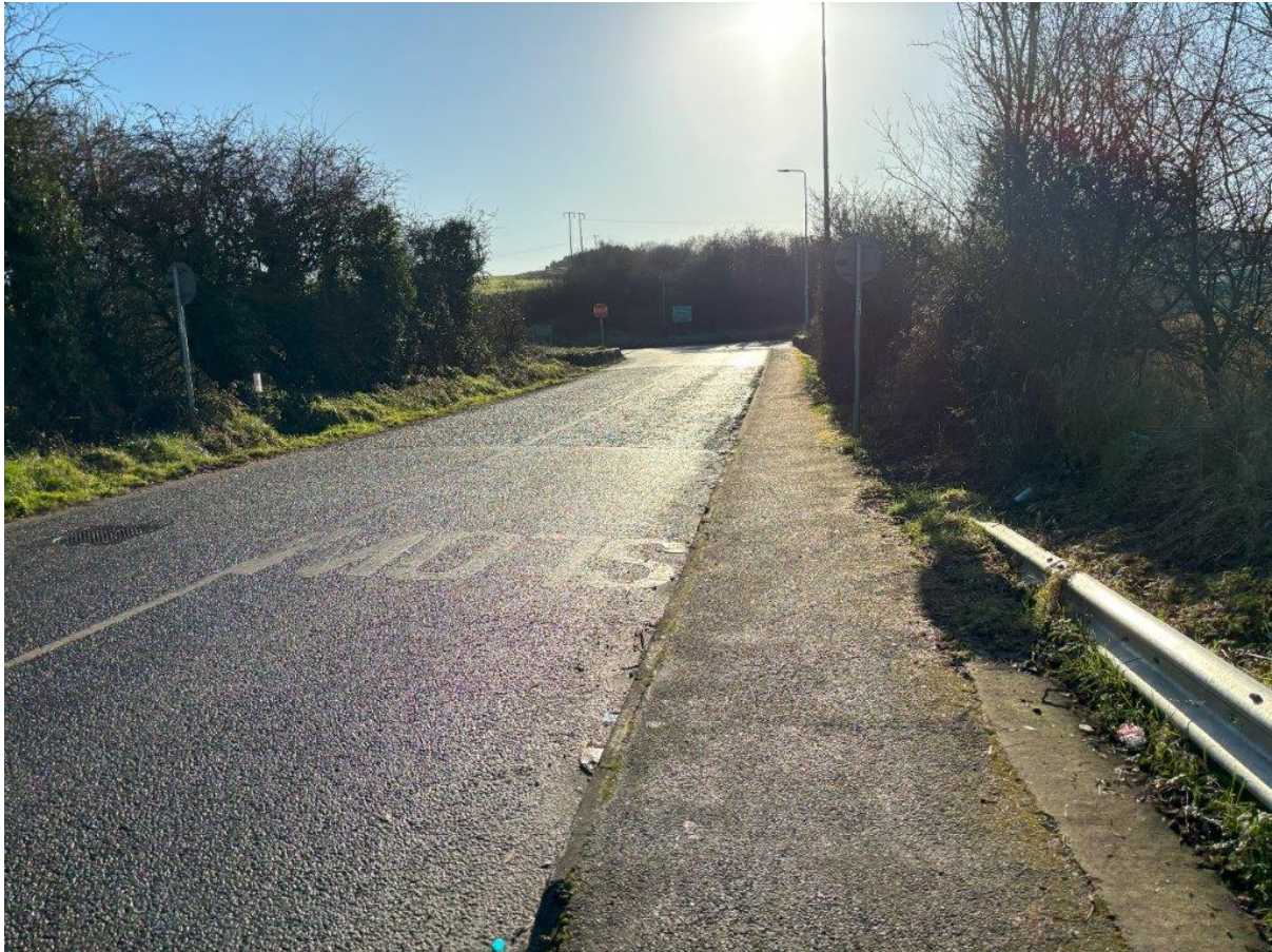
Photo 9 Approach to N72 junction from the L5331 (looking southwards)
