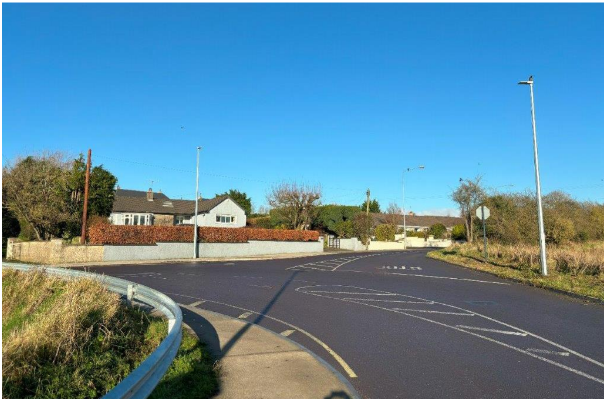
Photo 8 Local junction off the L5331 north of the proposed N72 works (looking northwards)
