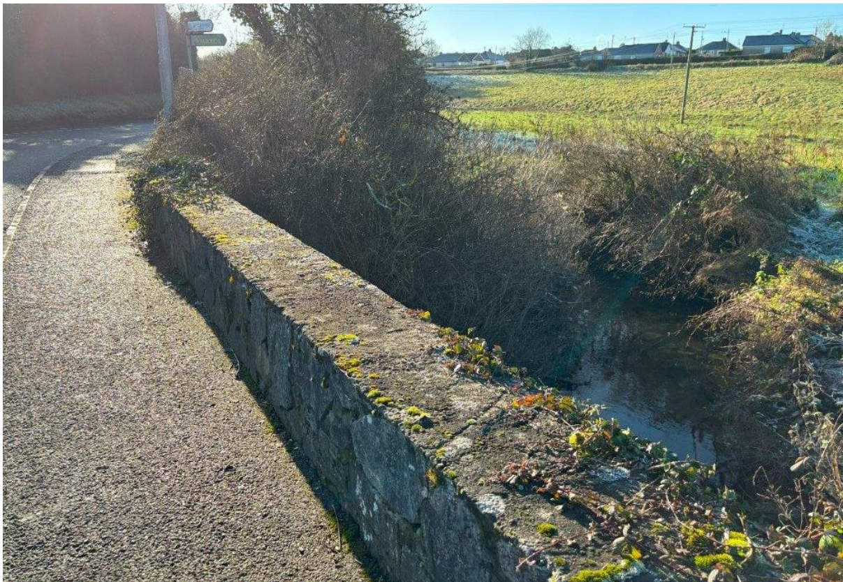
Photo 10 Existing bridge/culvert Parapet wall on the L5331 (looking southwards)
